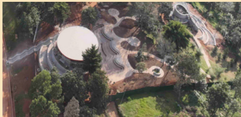
Figure 35. Paul's Glade and Mausoleum at 87% construction completion
