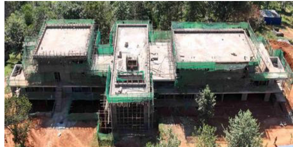
Figure 34. The Ubuntu Global Faculty Centre at 49% construction completion
