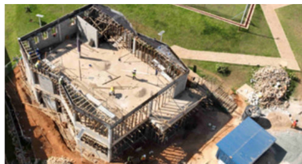
Figure 36. The New Recreation Centre at 45% construction completion
