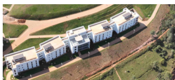
Figure 32. Student Accommodation Facility (Cluster 8)
